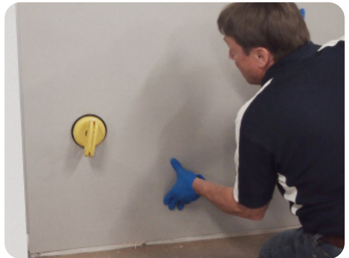
Use suction cup to fix panel.
