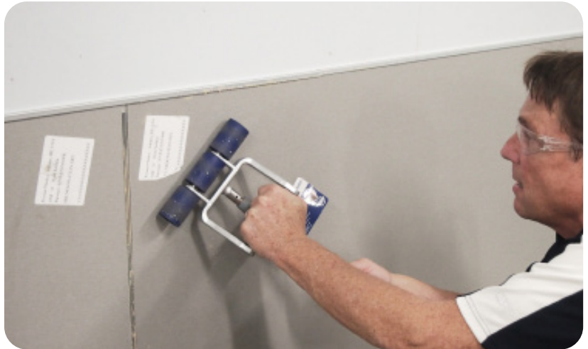
Roll with D-handle laminate roller.
