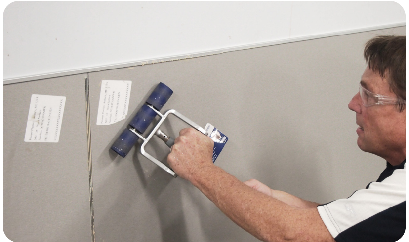
Roll with D-handle laminate roller.
