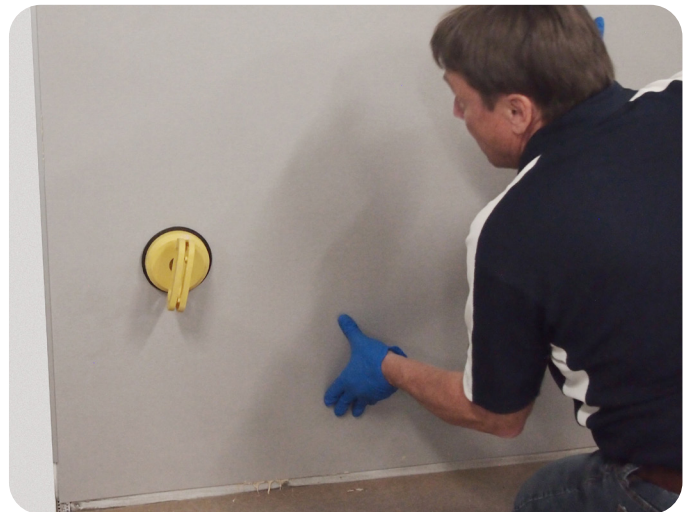
Use suction cup to fix panel.
