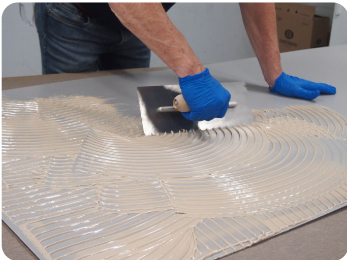
Use crosshatch method close to edge as shown in image above.
