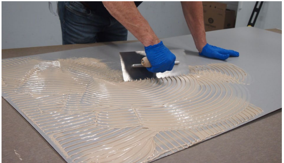
Use crosshatch method close to edge as shown in image above.
