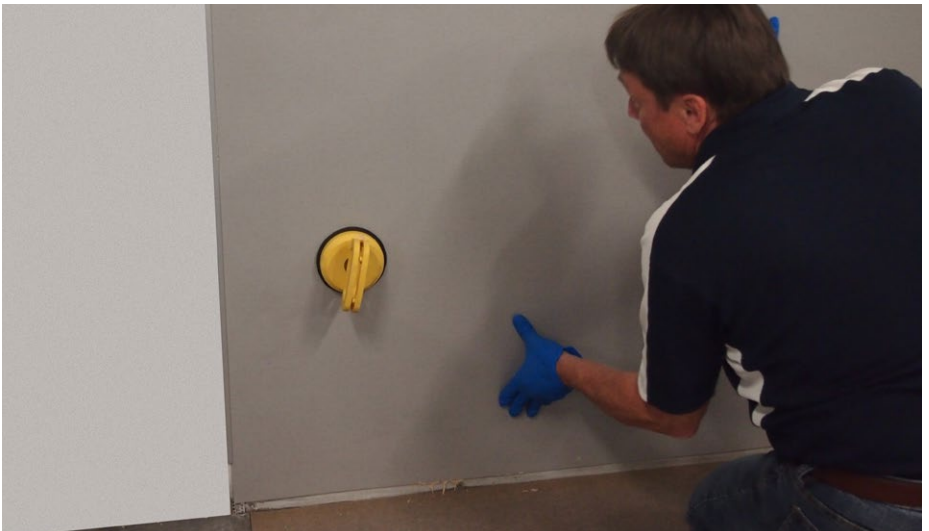
Use suction cup to fix panel.
