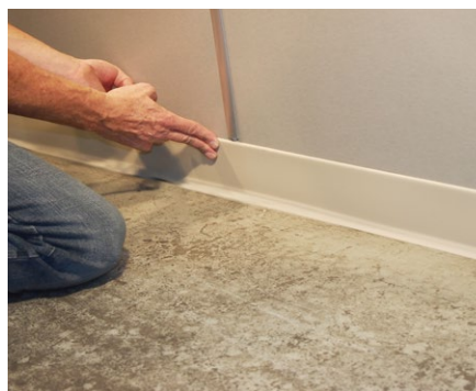
Use only flexible vinyl or rubber molding.
