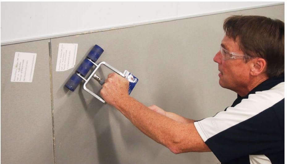
Roll with D-handle laminate roller.
