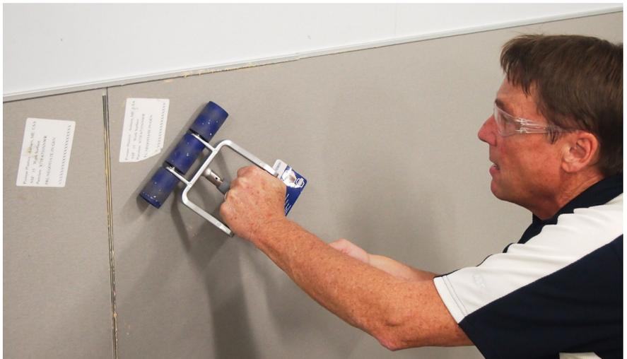
Roll with D-handle laminate roller.
